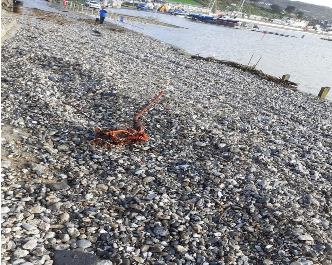
Stone and wave action also exposed the power cable that supply's all the Cobb buildings
