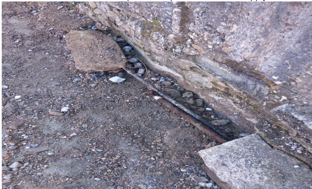
Stone and wave action also exposed the power cable that supply's all the Cobb buildings
